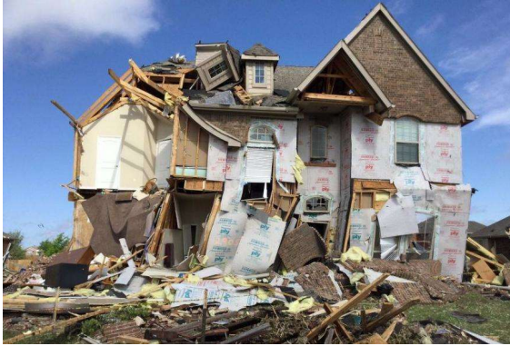
Poor load path
