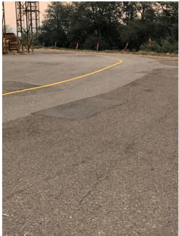
ROADWAY BETWEEN PLANT FIVE AND SIX
