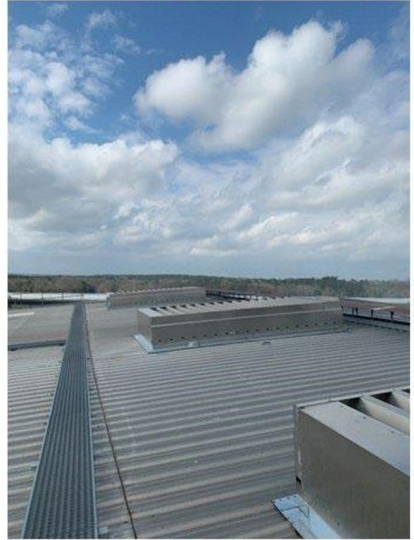
View of vent from rooftop
