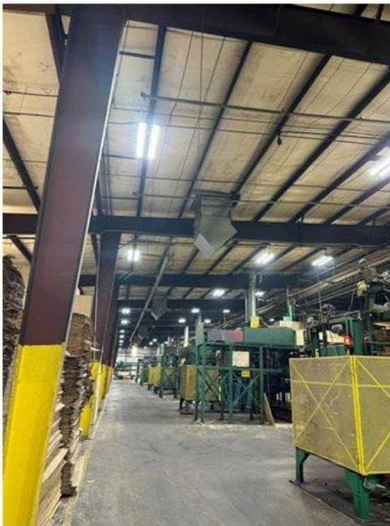
4 fans added on glue line
