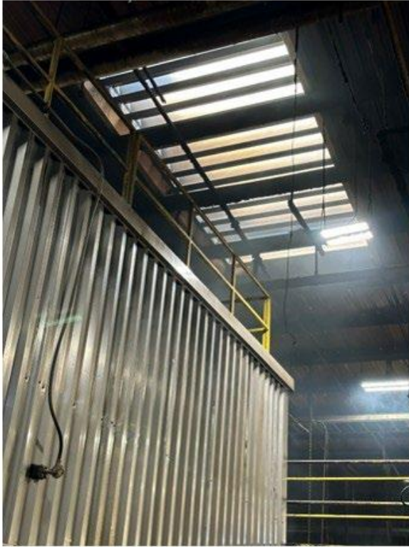
View of vent from inside
